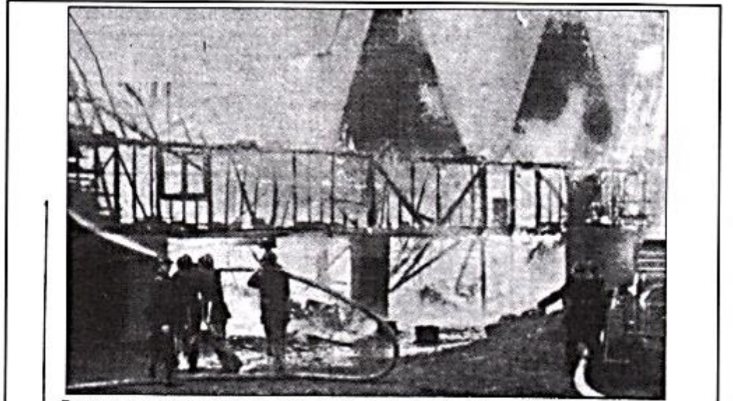
Damage amounting to £6,000 was caused by fire at Beagles Wood Farm, Pembury, on Friday last week.
